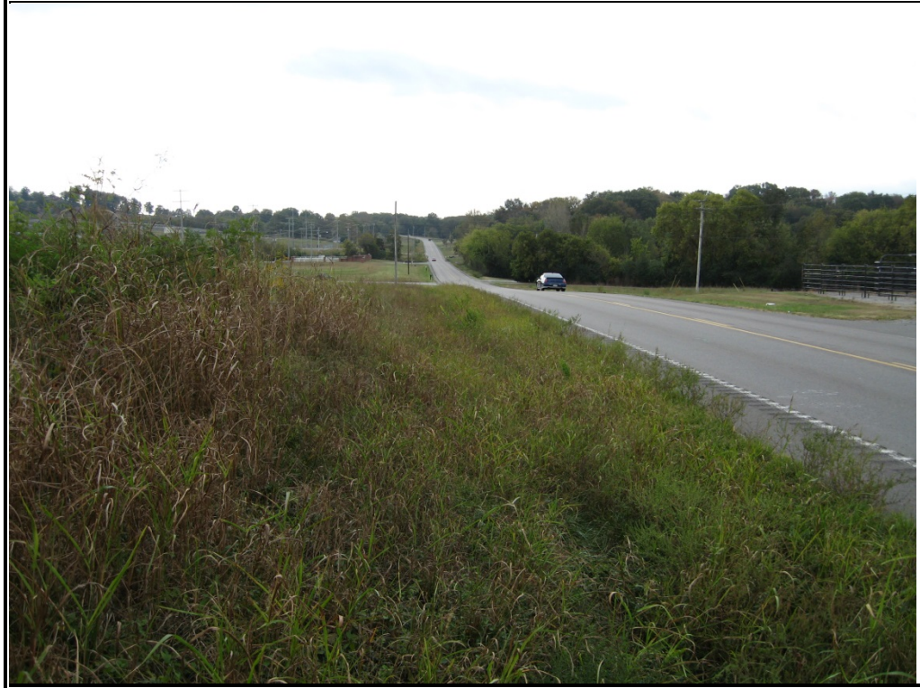
Photo: 4 By: M. Williams Date: 10 October 2014 Feature: Roadside Ditch
