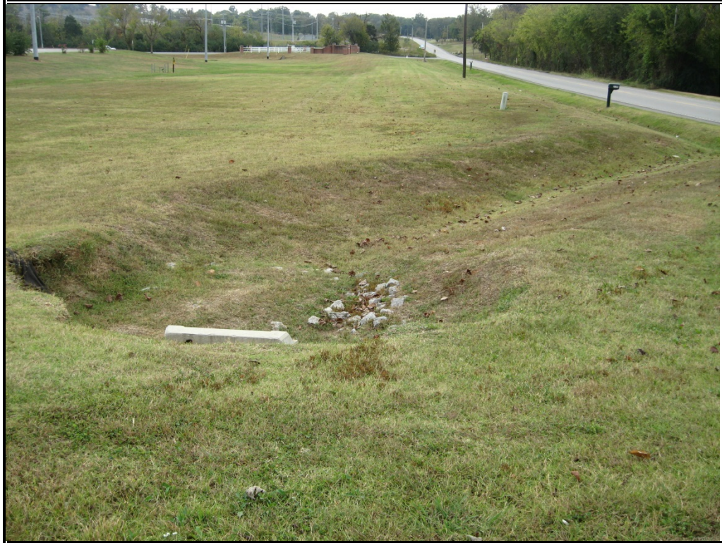
Photo: 6 By: M. Williams Date: 10 October 2014 Feature: Roadside Ditch
