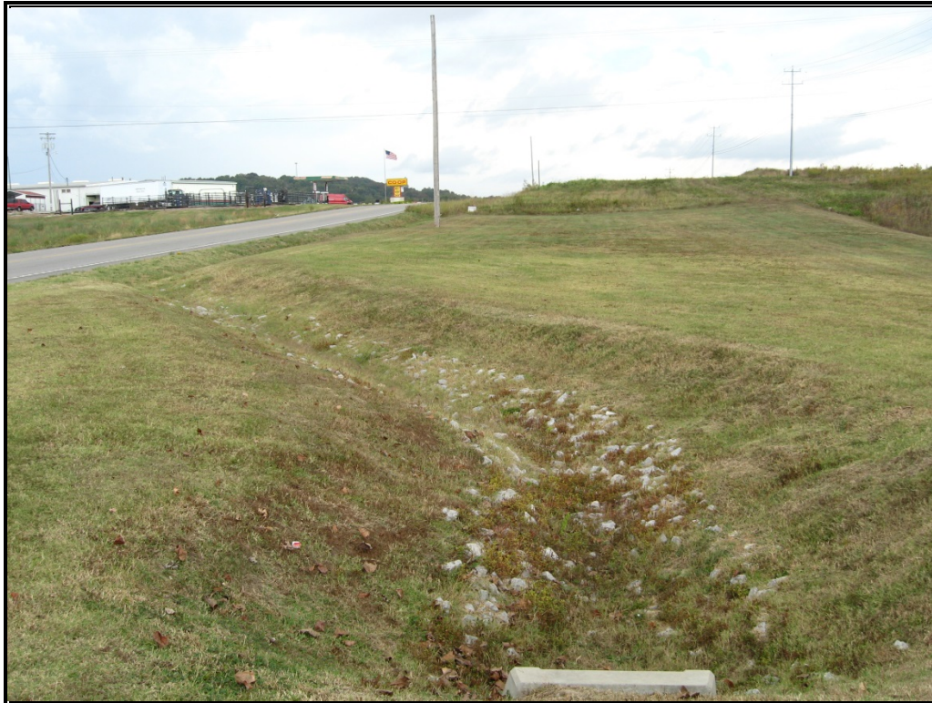
Photo: 5 By: M. Williams Date: 10 October 2014 Feature: Roadside Ditch
